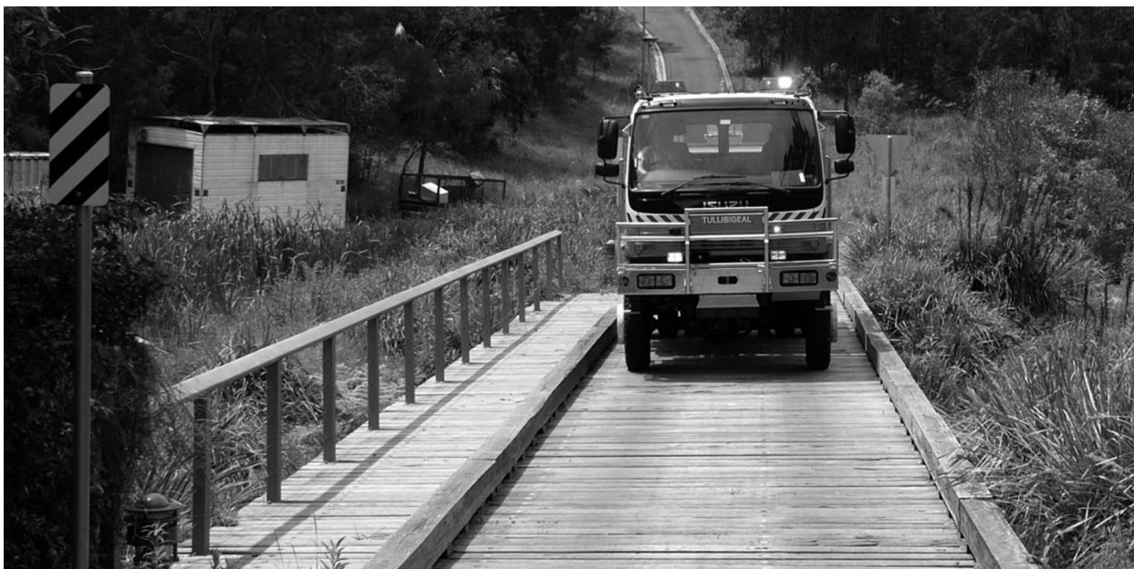
Property access should not restrict firefighting access. Bridge loadings should be clearly marked.
