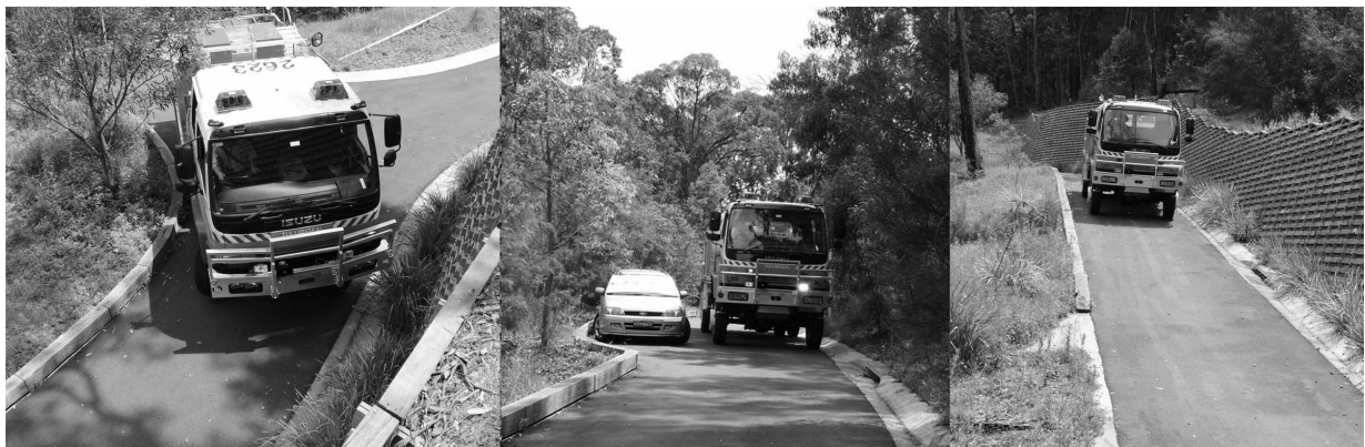
Examples of public road access arrangements that do not facilitate bush fire fighting.
