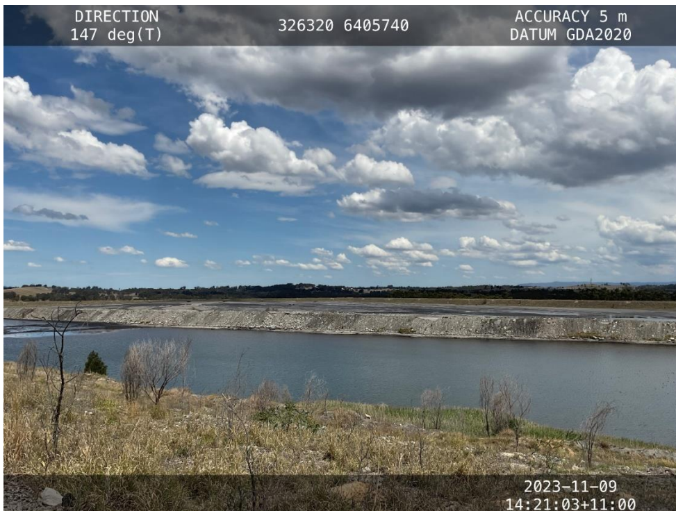
Plate 30: RCN Tailings Dam 2.
