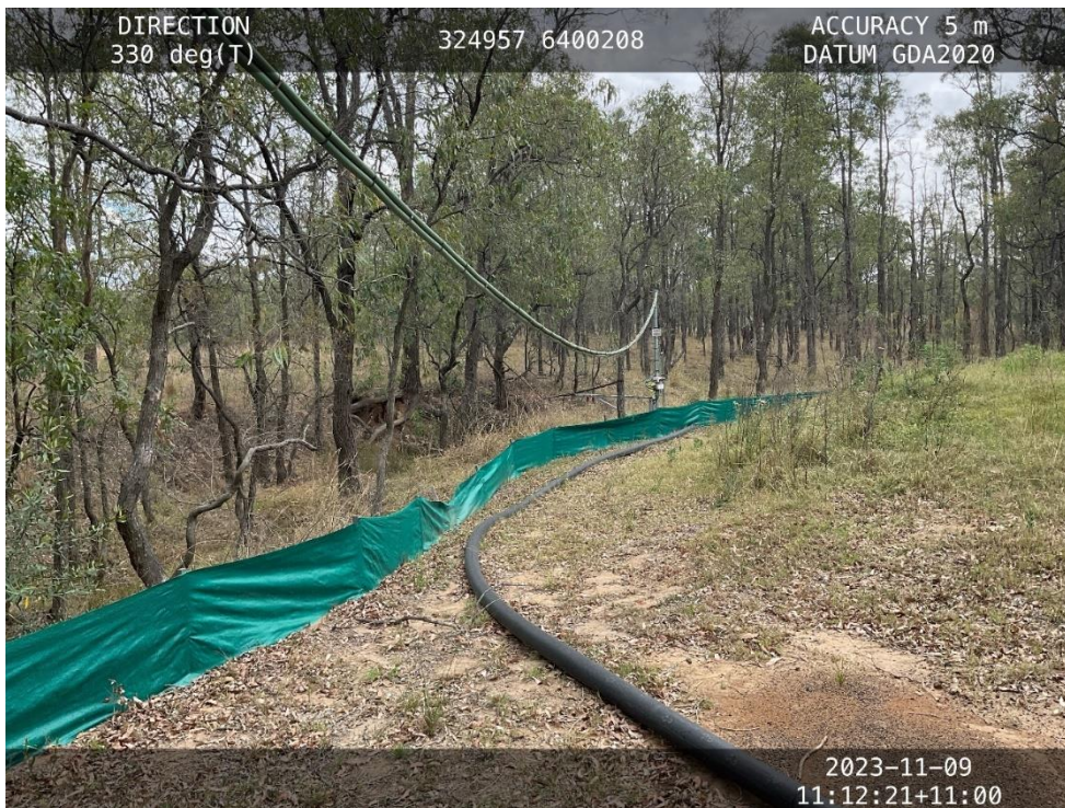
Plate 9: RCS Stonequarry Gully Sediment Fencing.
