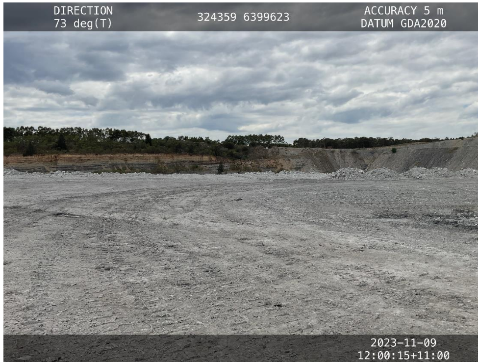
Plate 1: RCS Capping Progress of Tailings Emplacement Area 3.
