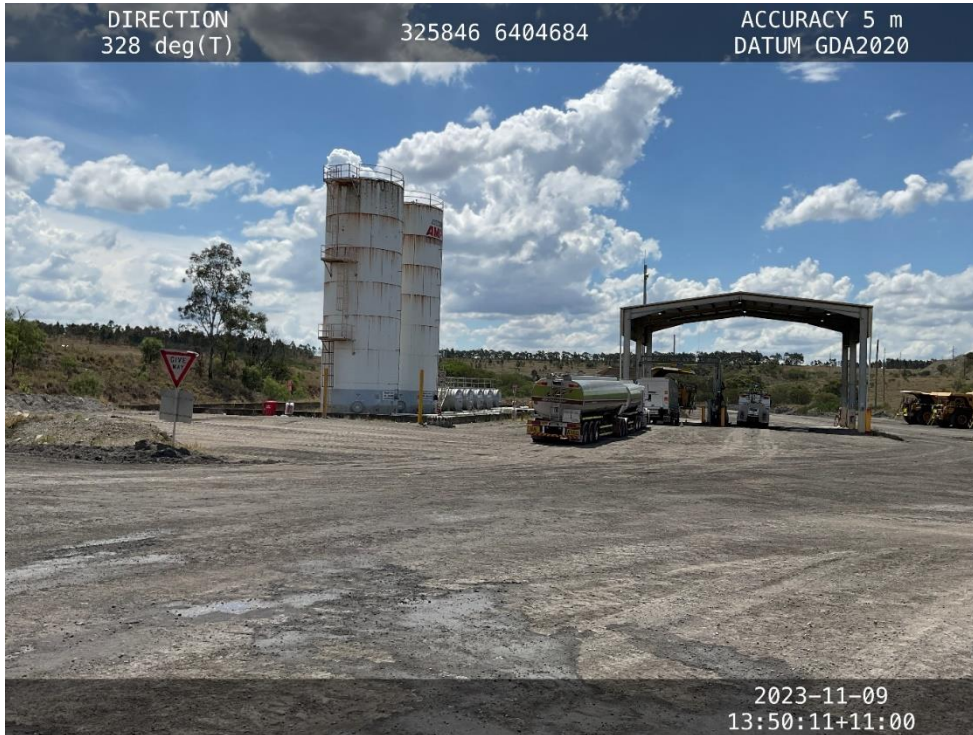
Plate 33: RCN Fuel Farm.
