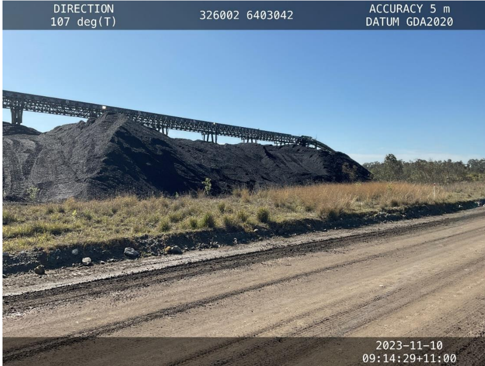
Plate 27: RCS Product Coal Stockpile adjacent to Train Load Out.
