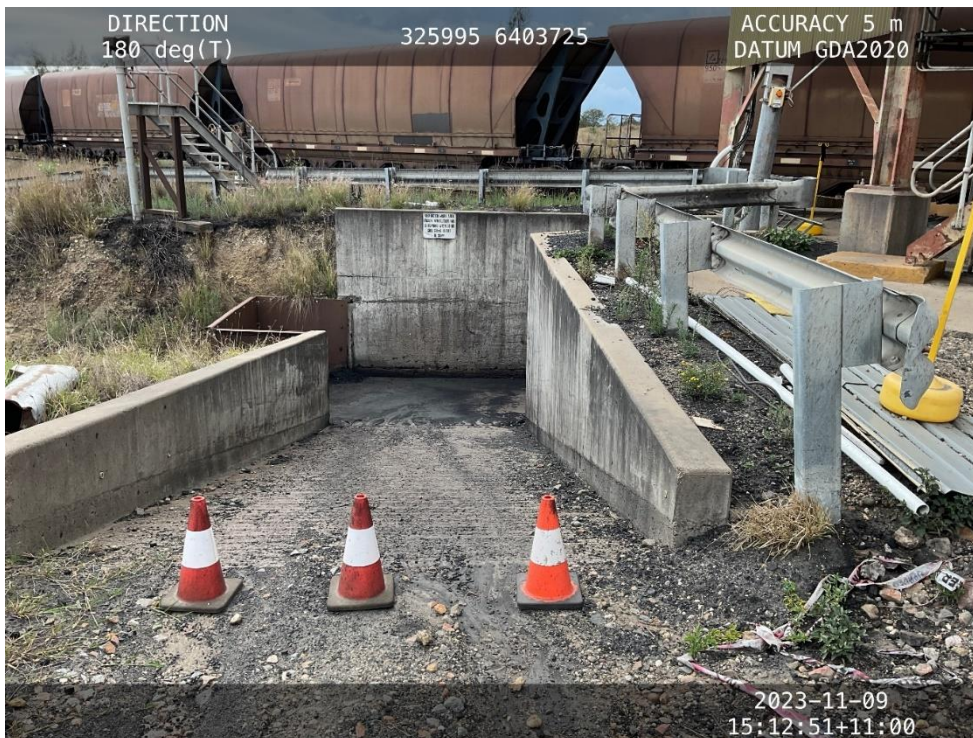
Plate 32: Train Load Out Containment Bund.
