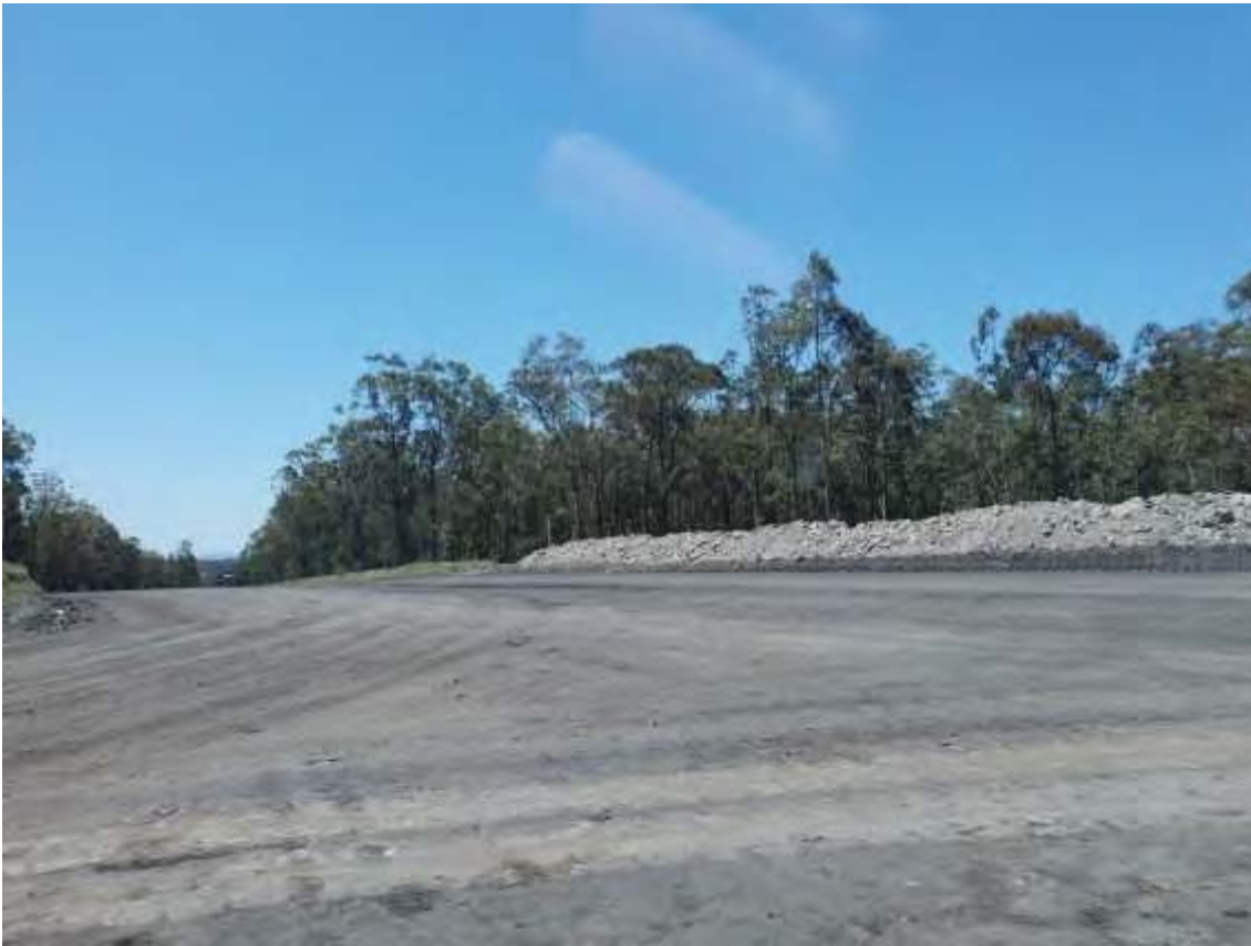
Plate 1 – Example of haul road (well maintained)
