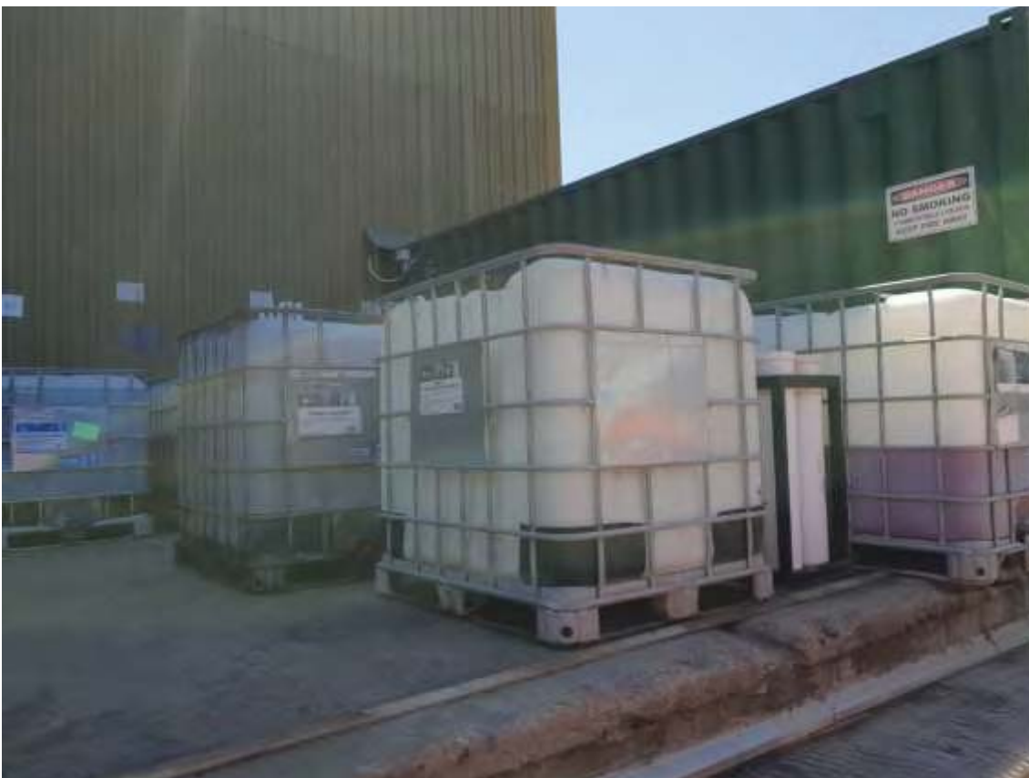
Plate 10 – Storage of chemicals within a hardstand bund
