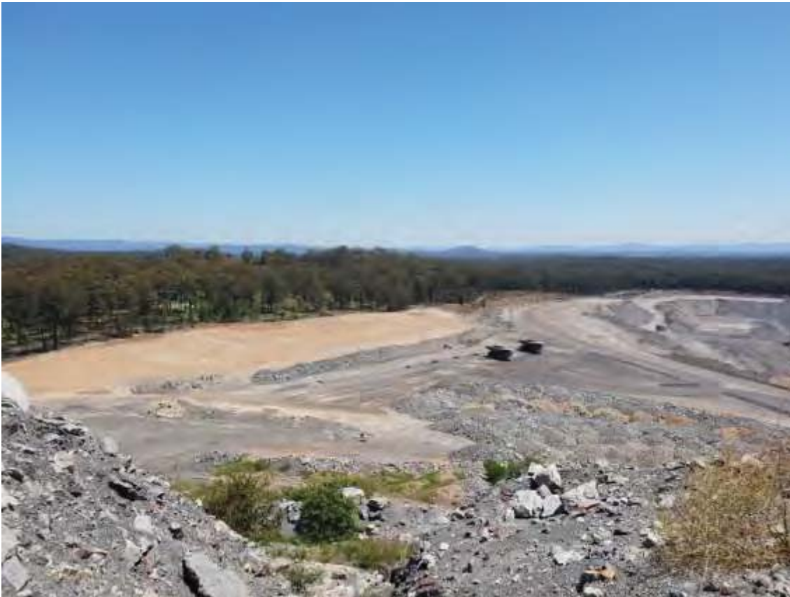
Plate 3 – Progressive establishment of final landform within the open cut
