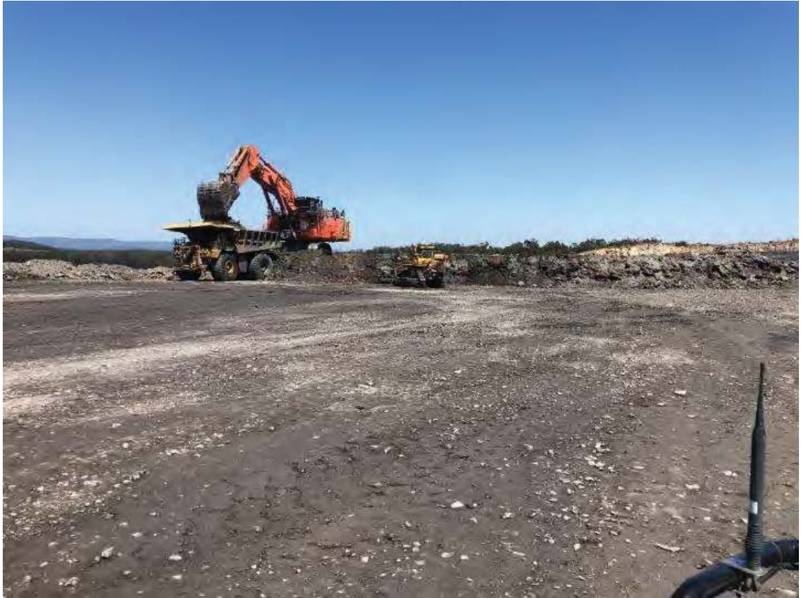
Photo 11: Excavator Mining Overburden
