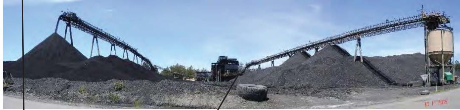
Bloomfield Coal Handling and Preparation Plant
