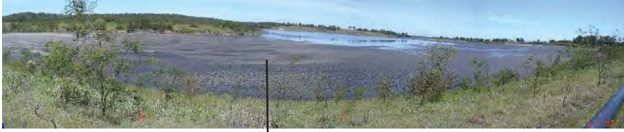
Bloomfield Tailings Dam
