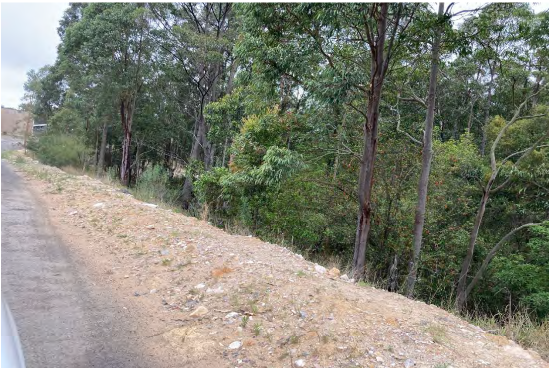
Plate 18 – Bunding installed on road surrounding rail loading facility
