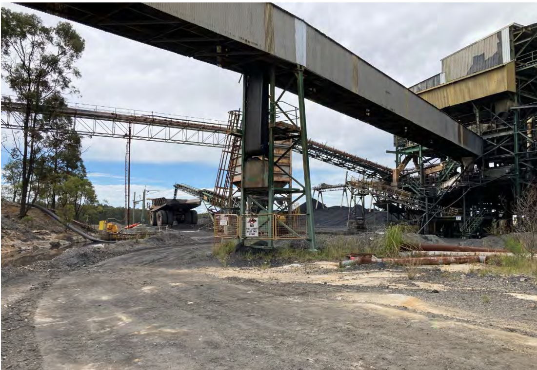
Plate 14 – Coal Preparation Plant Area
