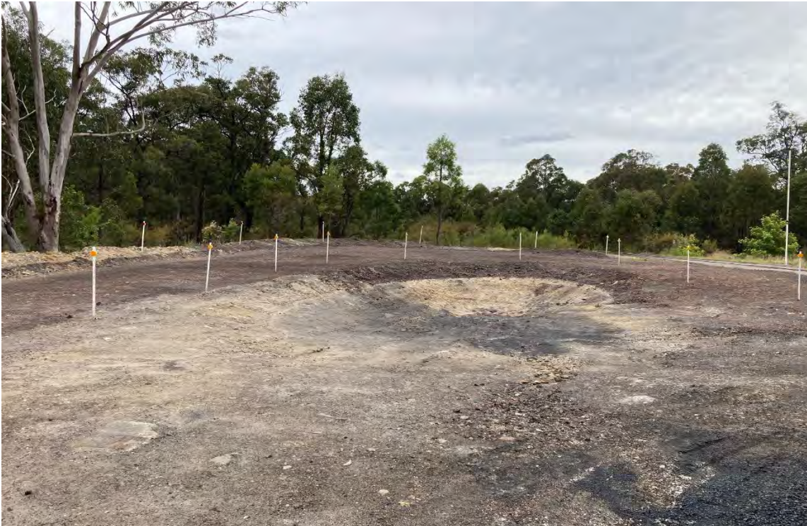
Plate 16 – Sediment basins installed around the rail loading facility
