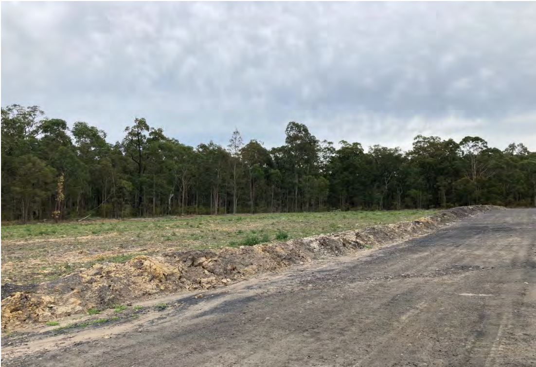
Plate 15 – Bunding installed around rail loading facility area
