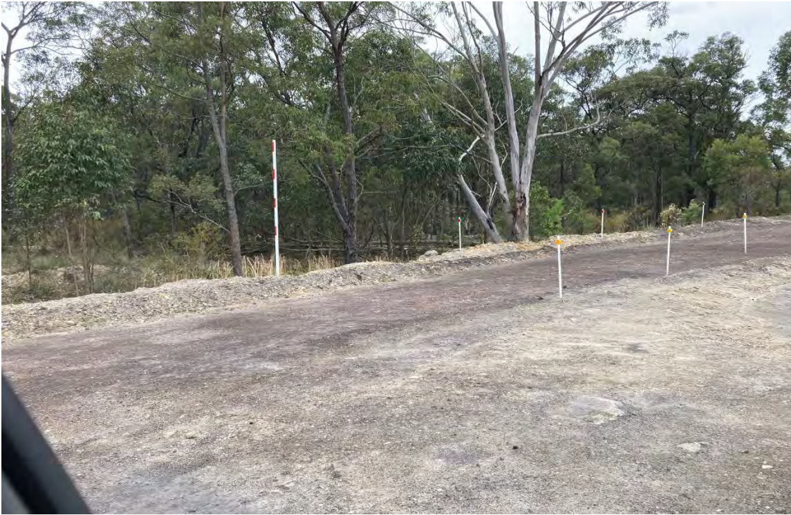
Plate 17 – Bunding installed on road surrounding rail loading facility
