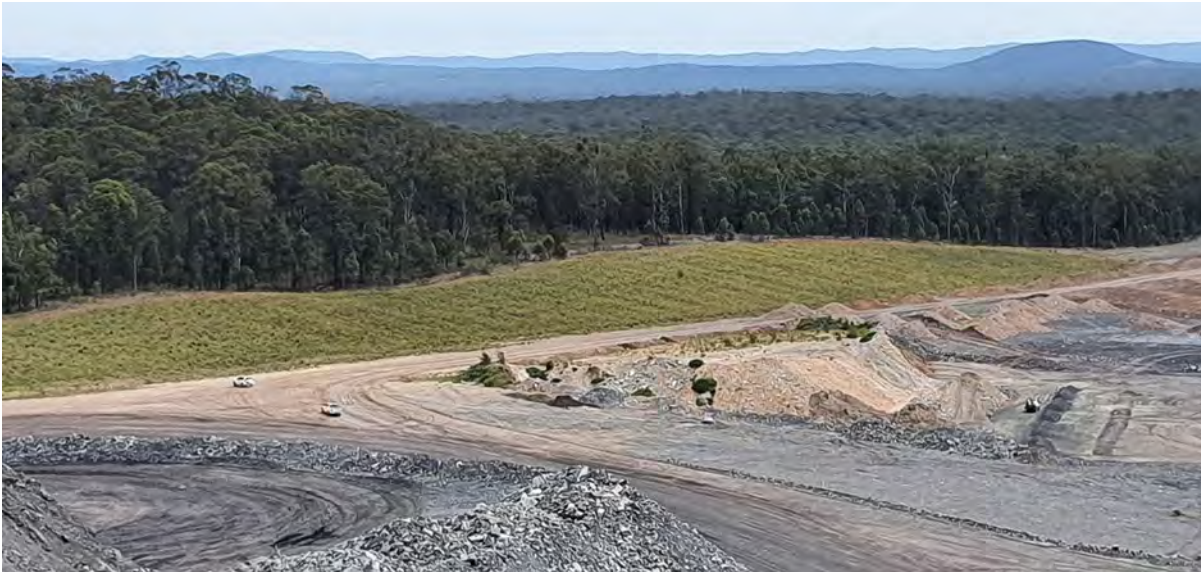
Plate 1 – S Cut Highwall Rehabilitation undertaken in 2020
