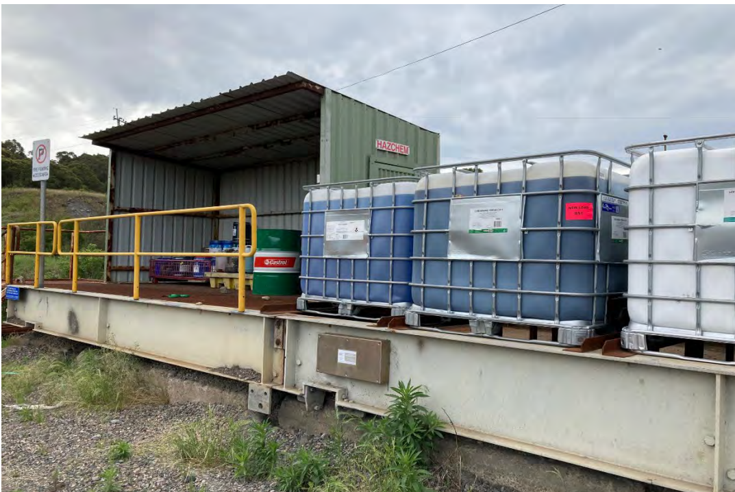
Plate 12 – Hydrocarbon storage facility
