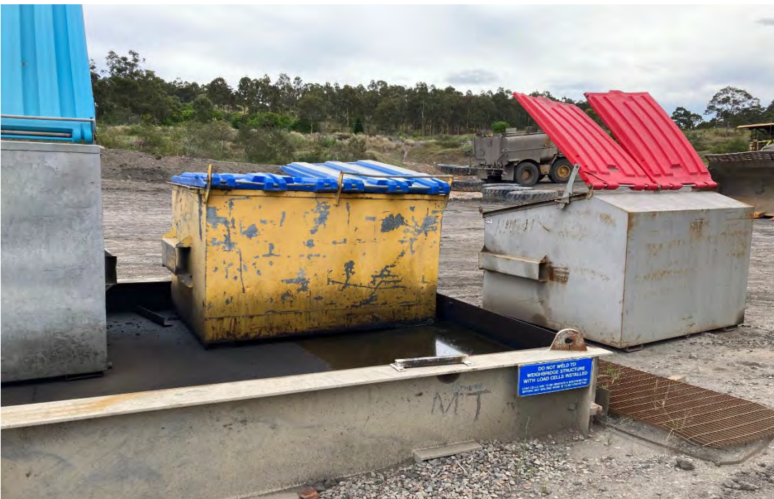
Plate 10 – Waste hydrocarbon containment area
