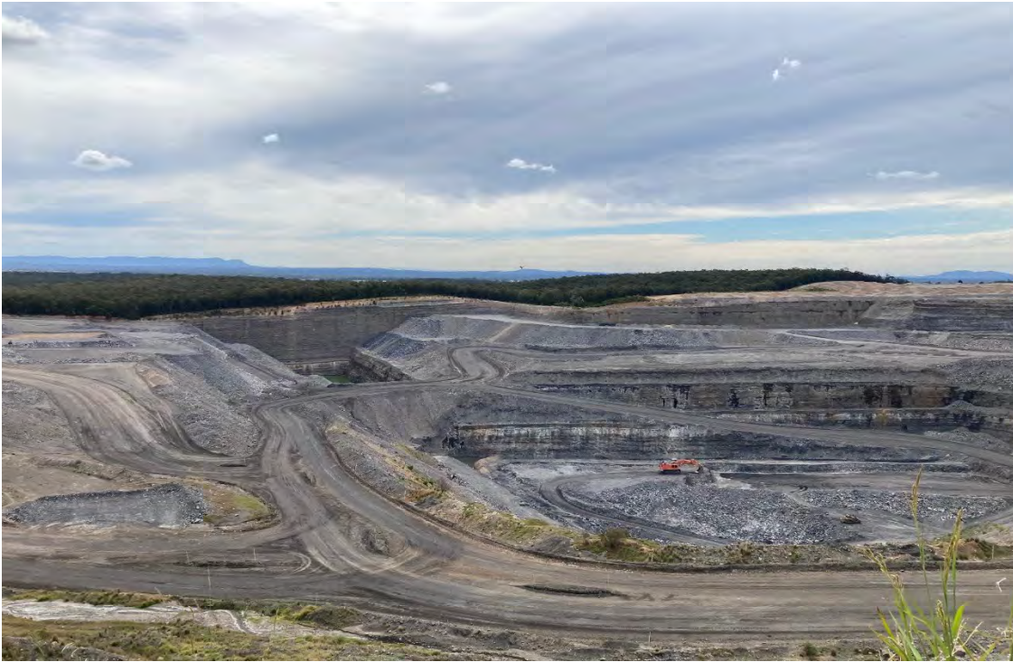
Plate 7 – Active Mining Area Open Pit “S” Cut
