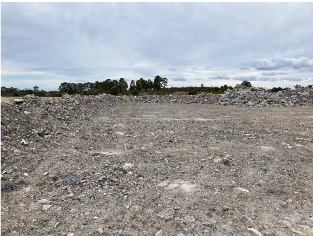
Plate 8 – Initial stage of capping on the tailings dam
