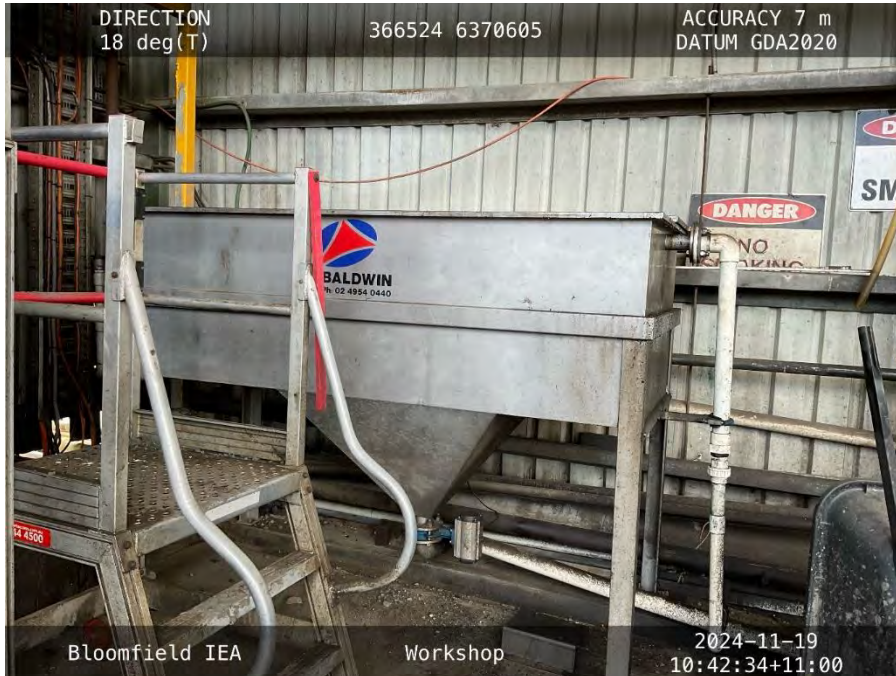
Plate 14: Oily water separator at workshop.
