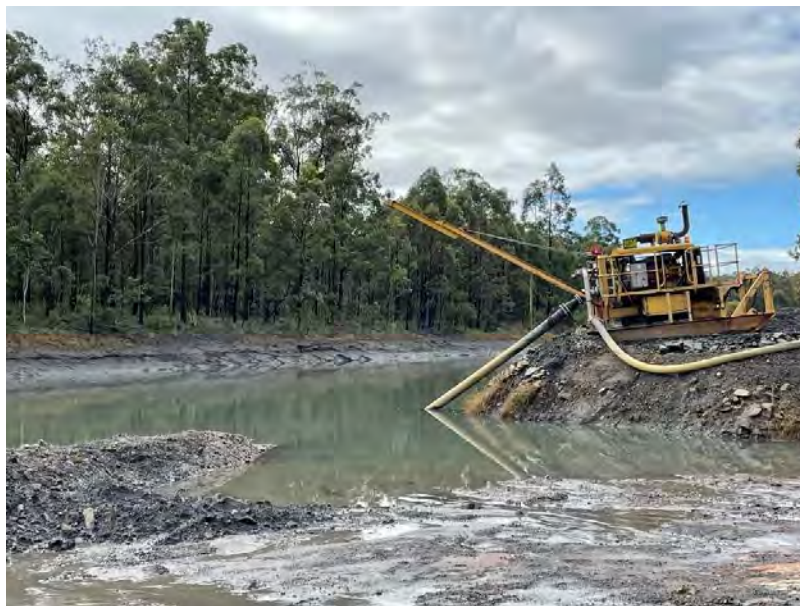
Photo 3 - One of the diesel pumps pumping water from the overland dam.
