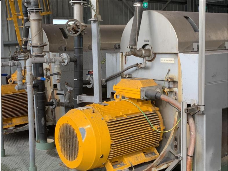
Solid bowl centrifuge at CHPP that produces dry tailings.
