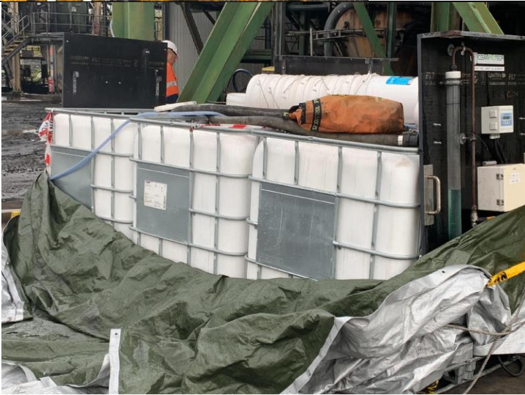
Banded flocculant with tarp cover blown off.
