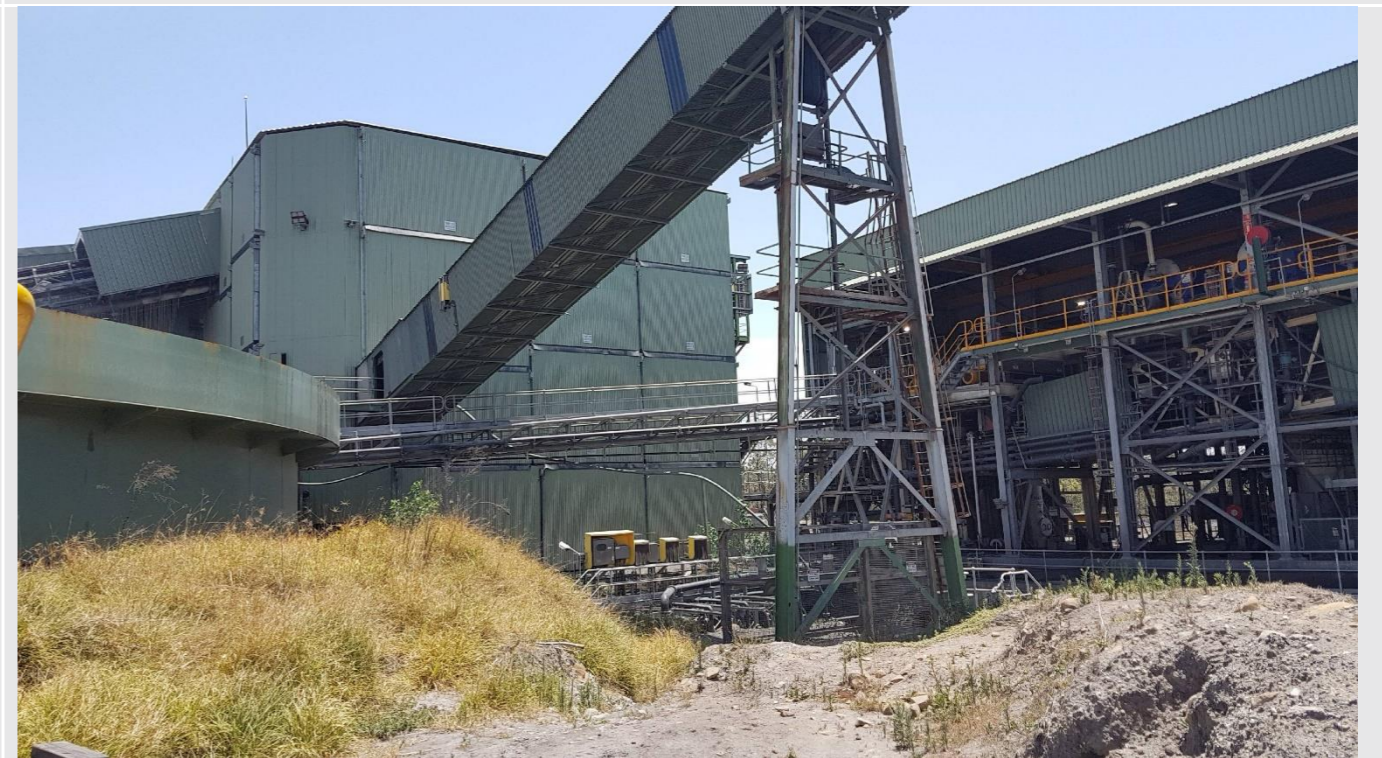
Plate 13 CHPP, showing noise walls added to the western side of the CHPP This has resulted in a 7 dBA drop in noise.
