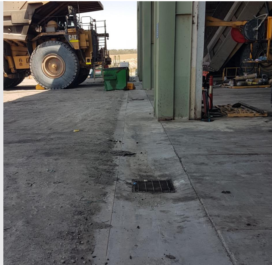
Plate 5 Dirty water drainage at the Mine workshop/refuelling bay
