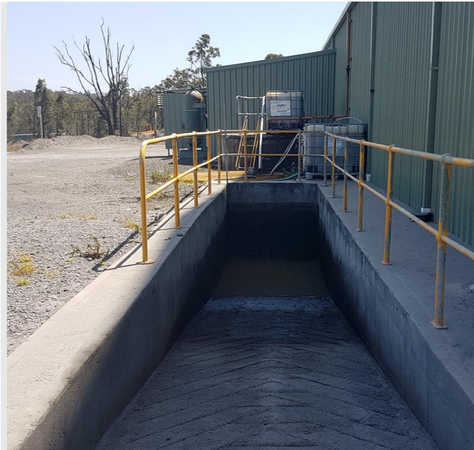
Plate 6 Oil water separator system
