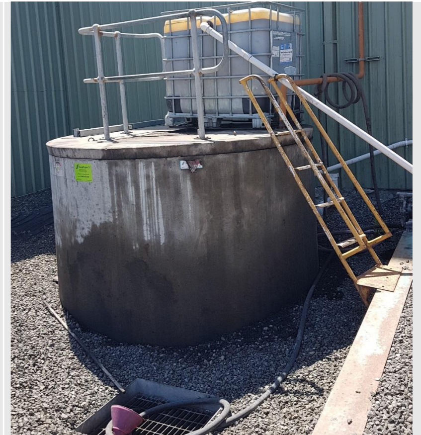
Plate 7 Oil water separator system, with drainage infrastructure for overflows
