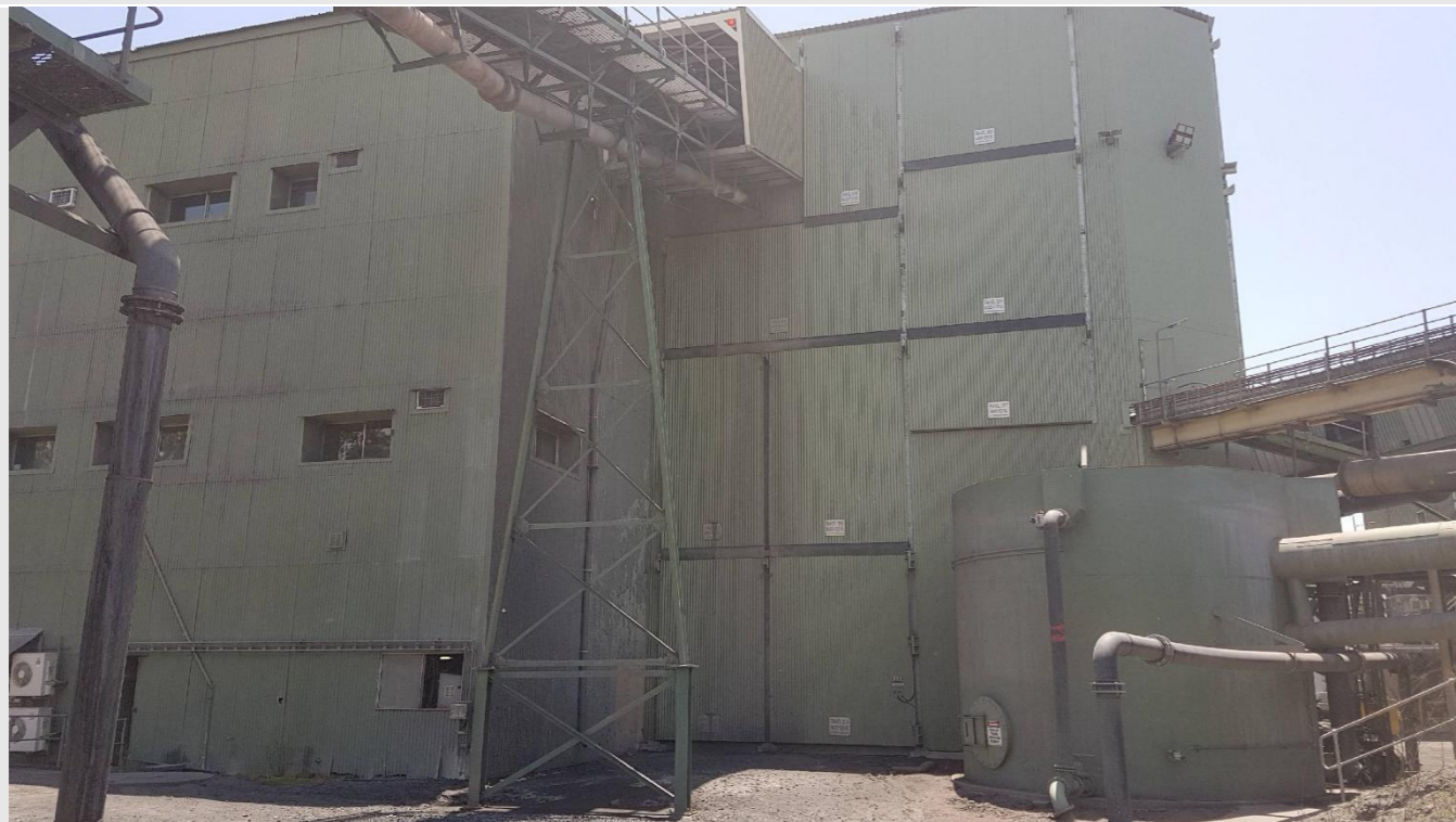
Plate 12 CHPP, showing noise walls added to the southern side of the CHPP This has resulted in a 7 dBA drop in noise.
