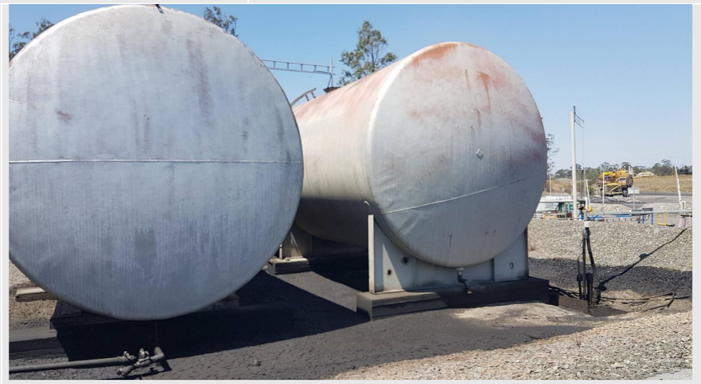
Plate 9 Above ground diesel storage tanks with clay liner bunding near the Mine entrance
