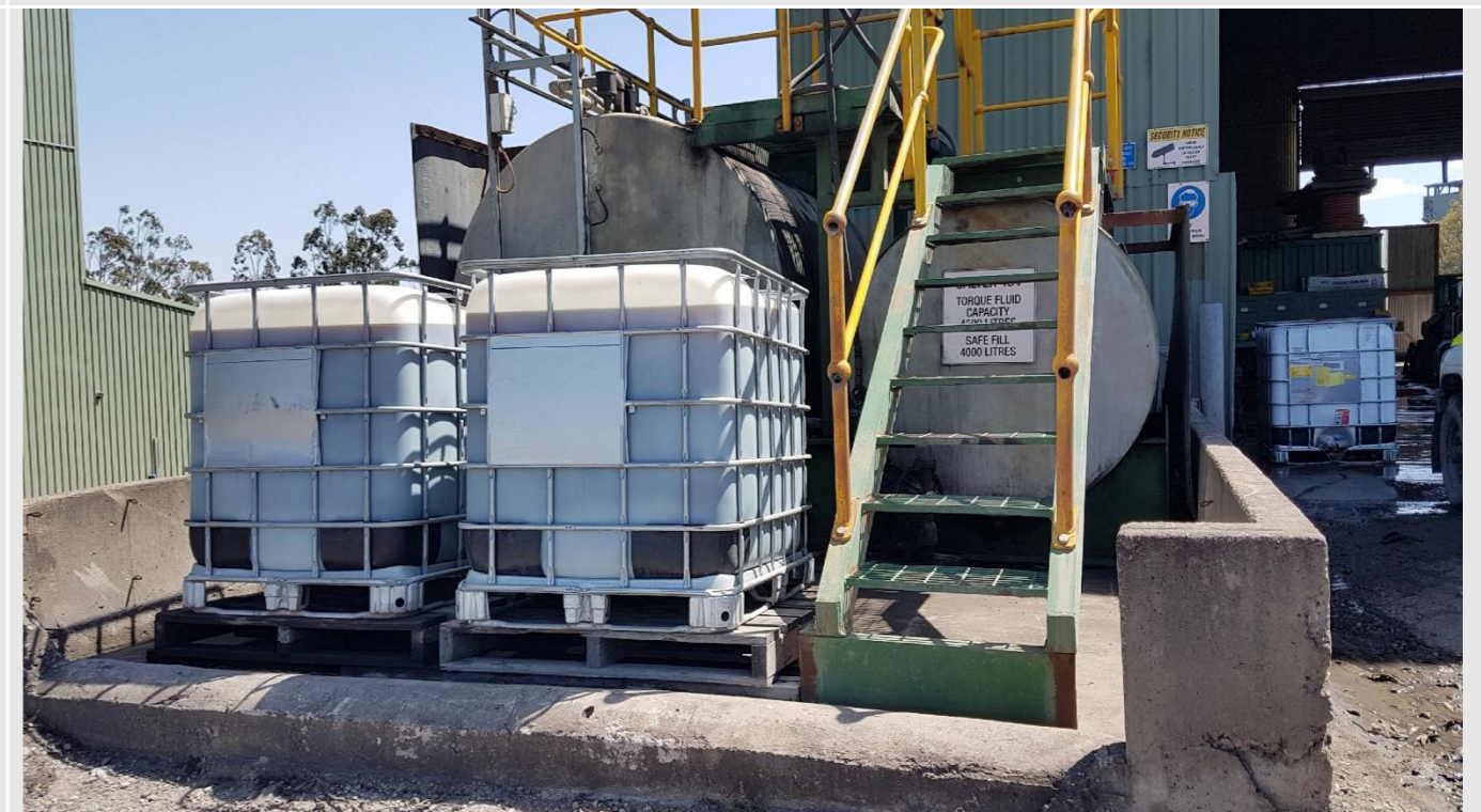
Plate 4 Above ground storage tanks with bunding outside workshop building
