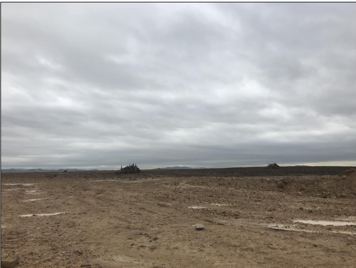
Plate 2 – Shaped and topsoiled rehabilitation with habitat timber ready for seeding
