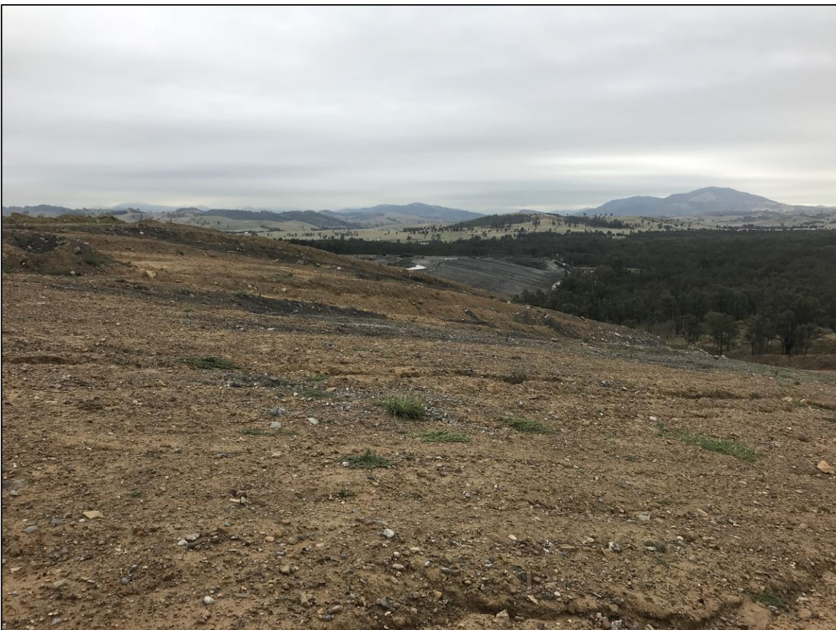
Plate 4 – Shaped area of Rehabilitation in Falbrook Pit ready for topsoil and seeding
