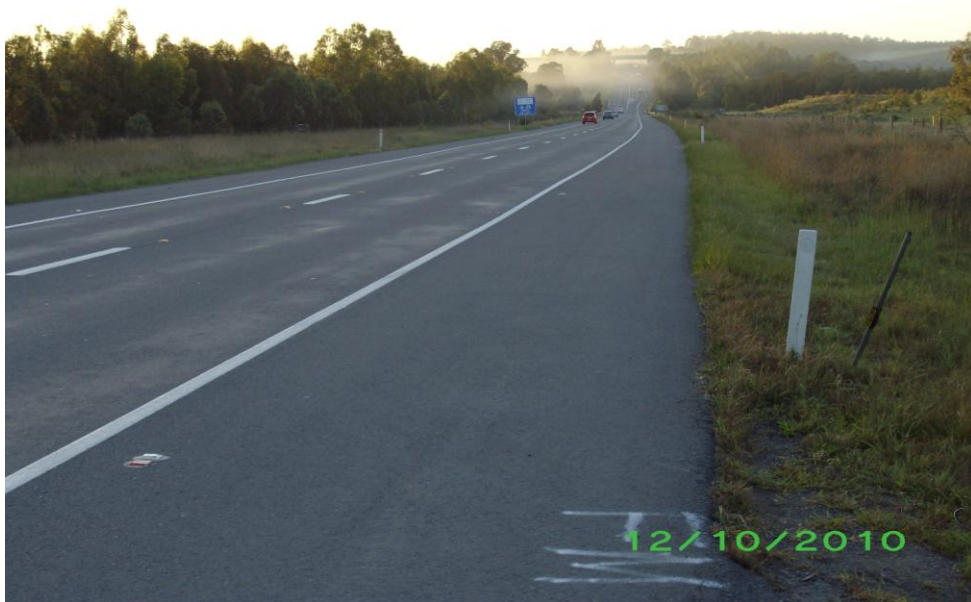
Figure 3 Photo looking south from compound access 1
