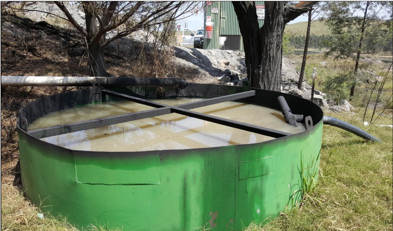
Plate 3 Oil water separator which had over topped
