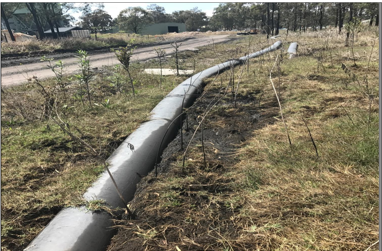
Plate 4 Hydrocarbon contamination behind workshop area
