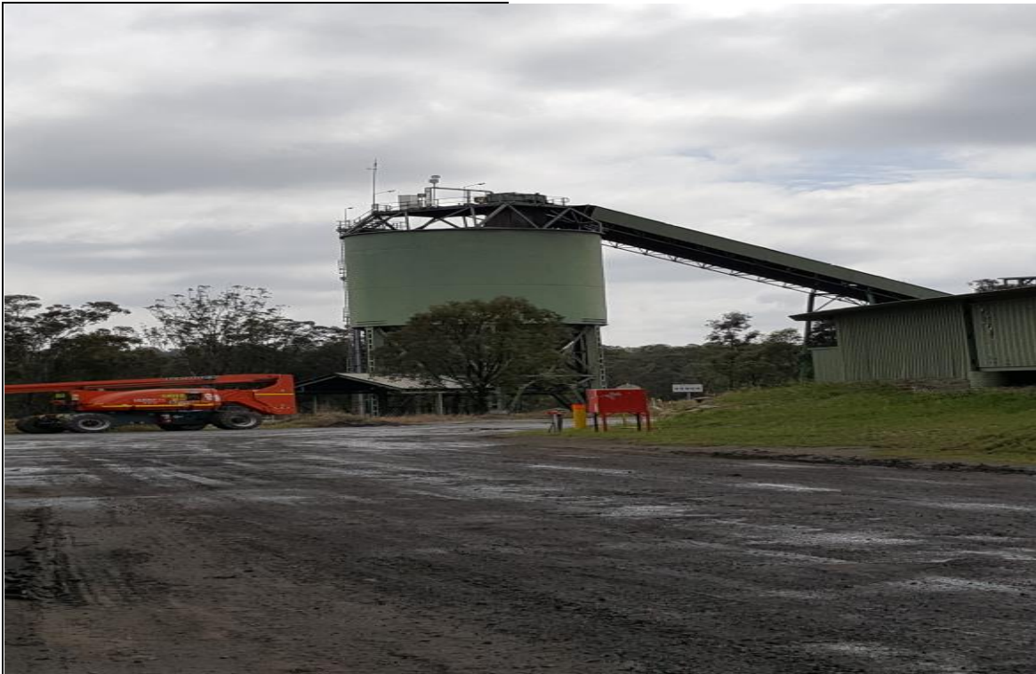
Plate 5 Cladding replaced on clean coal truck loading bin
