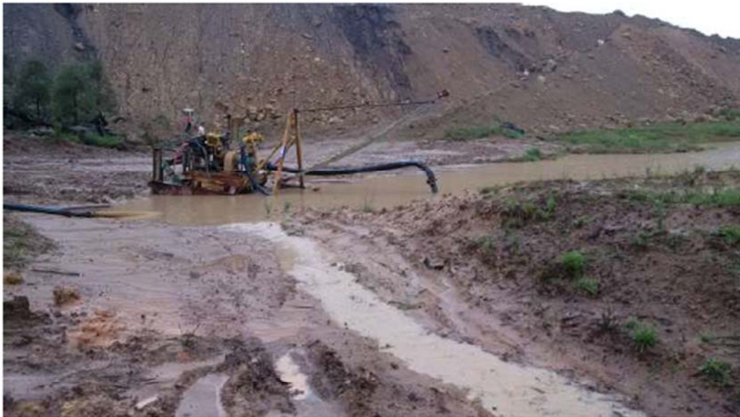
Photograph 3: West Pit out-of-pit-dump Sediment Dam (East).
