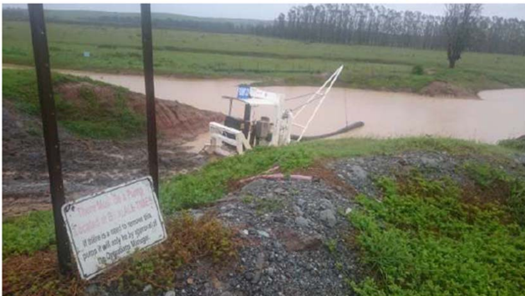
Photograph 5: Sediment Dam B5
