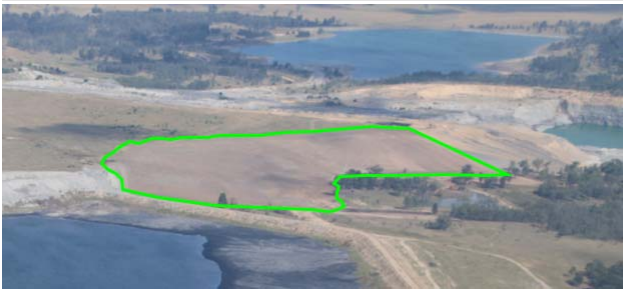
Plate. 8 Falbrook Pit – Stoney Creek Road batter rehabilitation facing west
