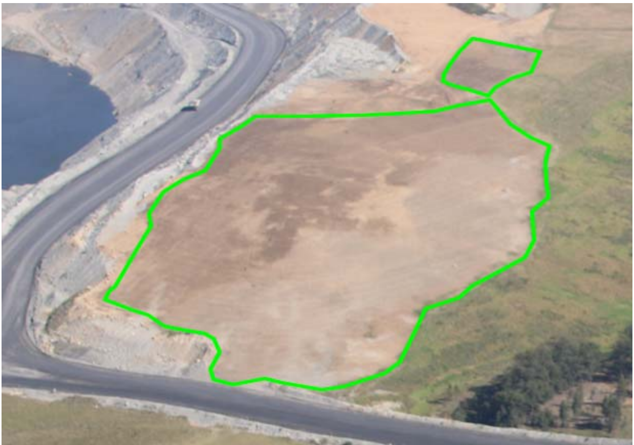
Plate. 7 Arties Pit dump facing north-west – photo taken while spreading topsoil over subsoil
