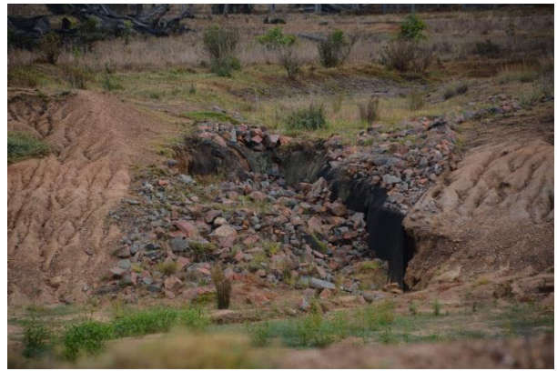
Plate 2 Erosion and Scour at Inlet to Dam B2 (Ref: E796B_074)
