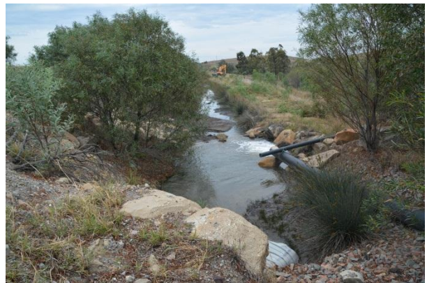
Plate 4 Dirty Water Drain Upslope of Clean Water Drain at "the cattle yards" (Ref: E796B_272)
