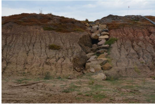
Plate 1 Erosion Scour from Road to Dam B5 (Ref: E796B_047)
