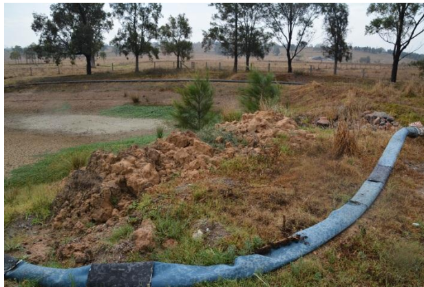
Plate 3 Sediment Placed on the Inside Wall of Dam B2 (Ref: E796B_066)
