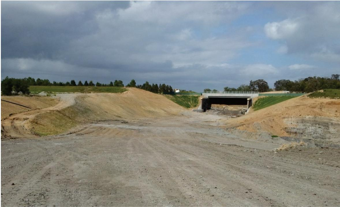
**Photo 4 - Tunnel under New England Highway. Note that batters have recently been hydro-mulched.**
