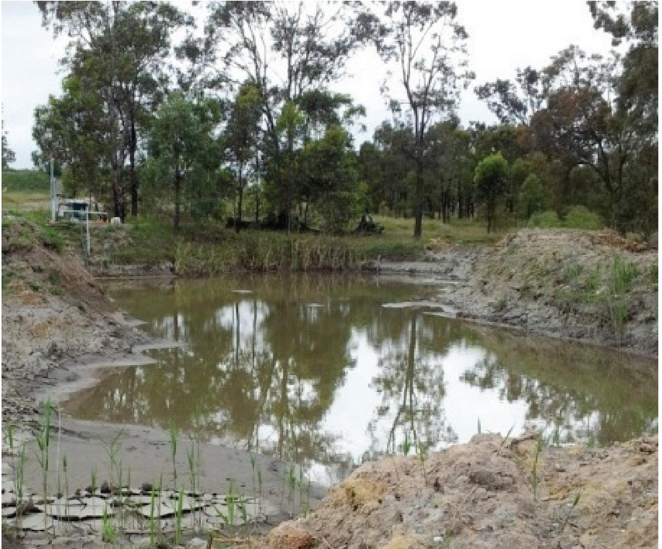
**Photo 6 Sediment Dam from collecting runoff from haul road with pump.**
